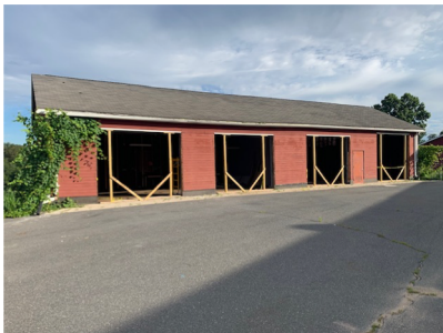
Storage Barn Repairs
